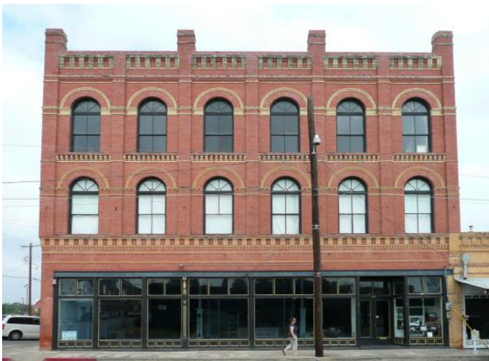
Masur Building (119 W. San Antonio St.)
