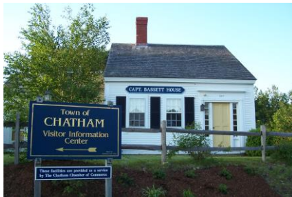
Capt. Bassett House Visitor Center
