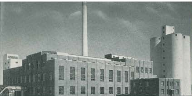
Amalgamated Sugar's Nampa facility newly constructed, circa 1942.
